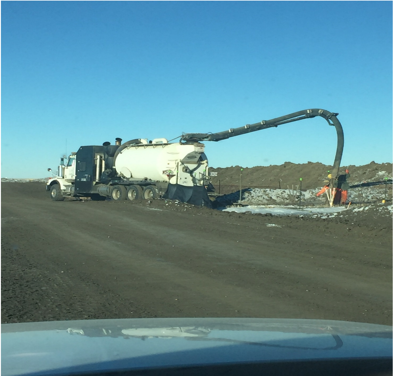
Hydrovac's locating existing lines before excavators come to trench.
