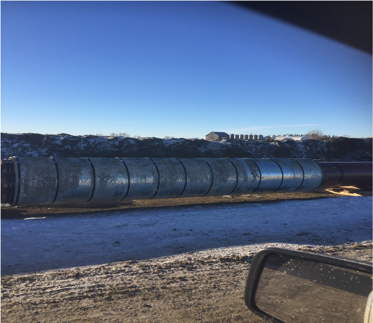
PIPE BEING PREPPED WITH CEMENT, TO BE LAID IN CREEK BED.
