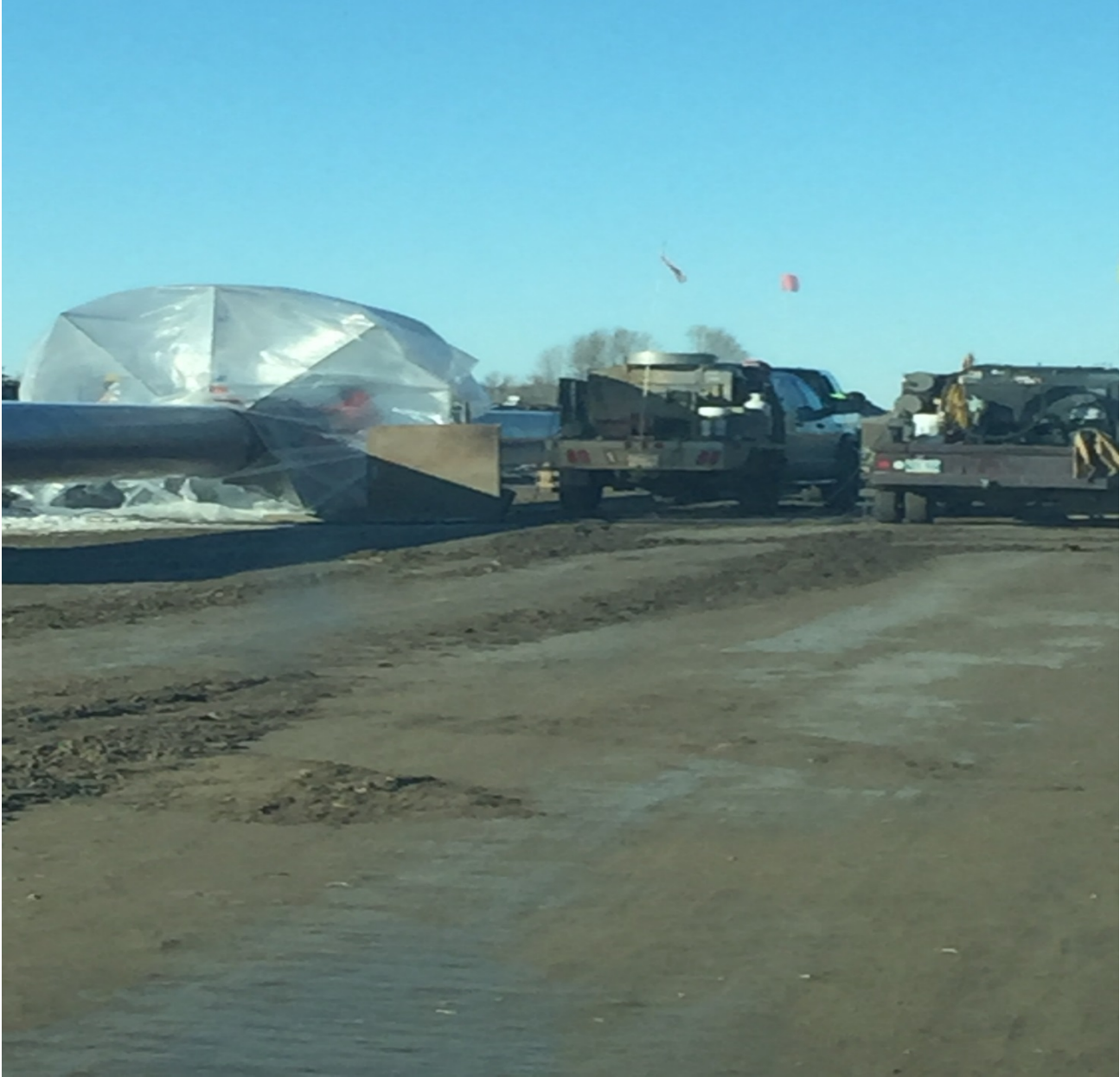
Welders working on pipe before tie-in crew arrives.
