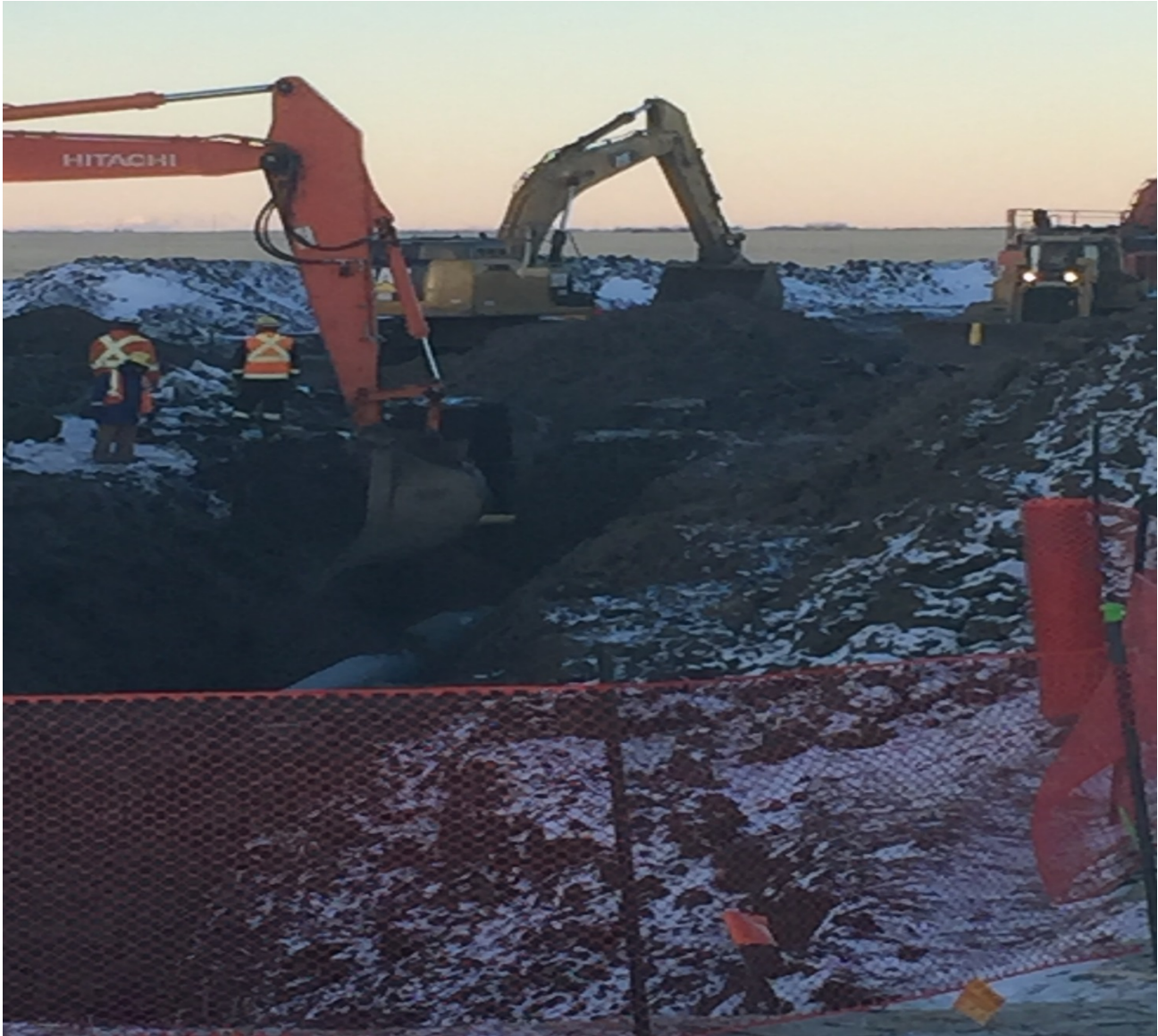
BACKFILLING PIPE AT ISKWAO CREEK
